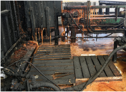
Water-based coating downstream – waste clean-up
