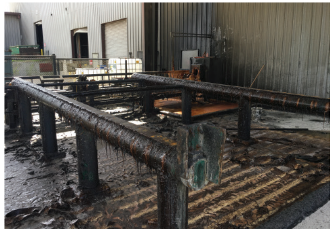
Further water-based coating mess during production
